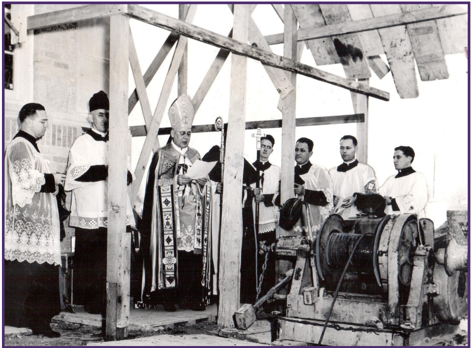
Laying of the cornerstone on addition to St. Anthony's Hospital on February 11, 1949 by Bishop Laurence J. Fitzsimon
