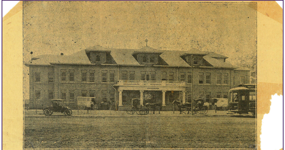
ST. ANTHONY'S SANITARIUM, AMARILLO, TEXAS.
